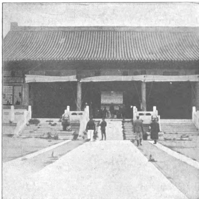
CH'EN-CH'ING GATE. Where Ministers alight from and take "Palace Chairs."
